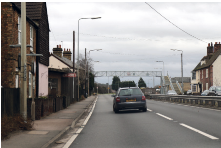
Photograph 9 – Biggleswade North - Sandy. Poor quality pedestrian environment, footways next to A1 route, pedestrian bridge unsuitable for vulnerable road users, segregation caused by A1.
